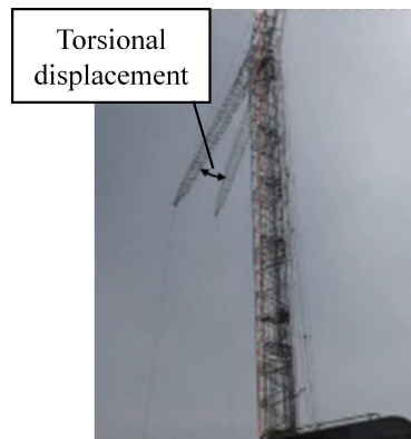
FIGURE 2. Torsional displacement of a tower
